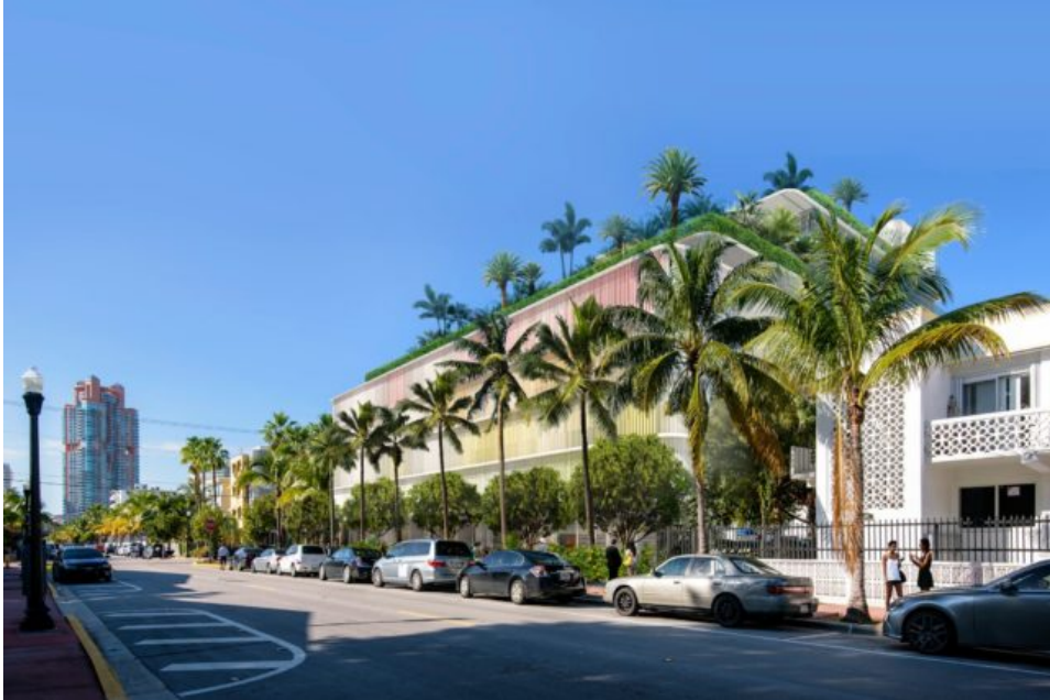
The garage will sit on top of a high-end restaurant and below a coterie of condos. (Courtesy Brandon Haw Architecture)
